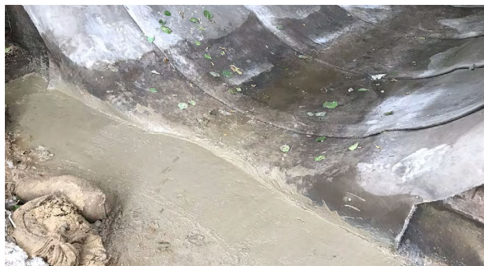
Leading edge buried in anchor trench
