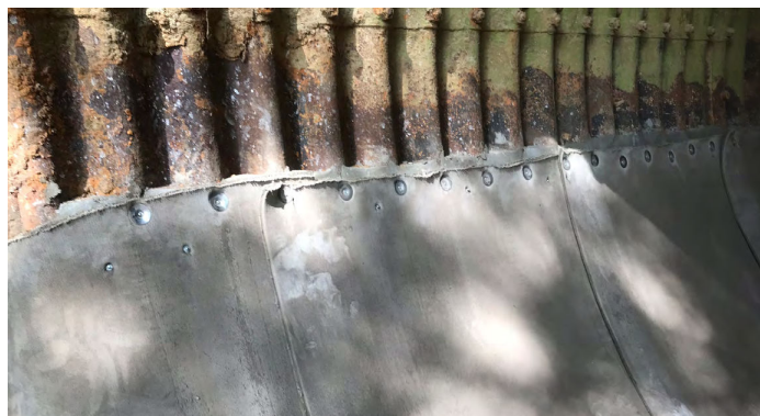
Perimeter edge secured with anchor fasteners and washers
