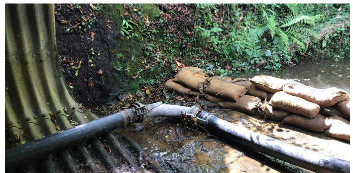
Sandbagging and pumping to dry the culvert for install
