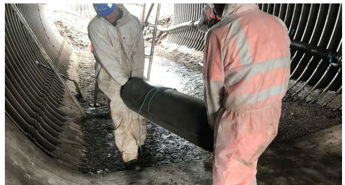
Bespoke batched CC transported into culvert
