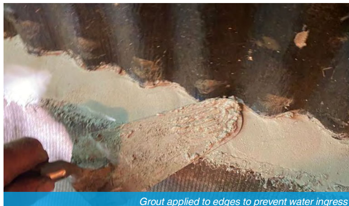
Grout applied to edges to prevent water ingress
