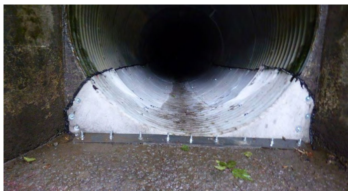
Trailing edge secured to concrete apron
