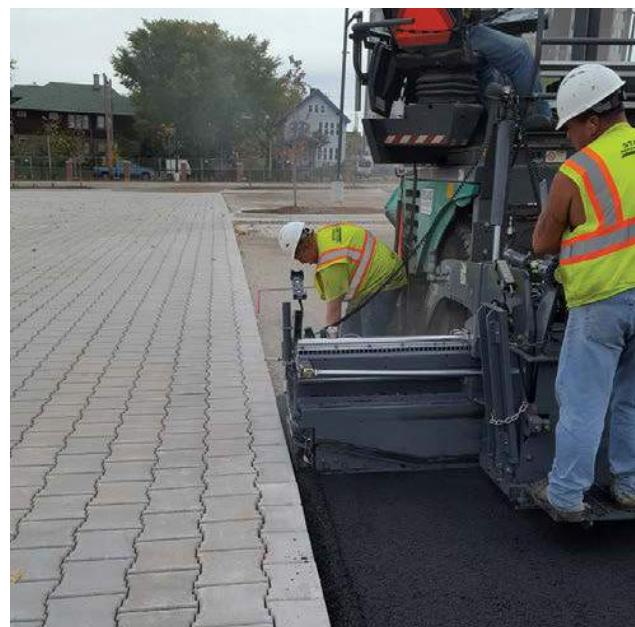
PaveDrain blocks work with existing infrastructure and can be used as the form for concrete or asphalt pours. Half blocks and end blocks square off corners eliminating cutting AND small pieces that are easier to dislodge.
