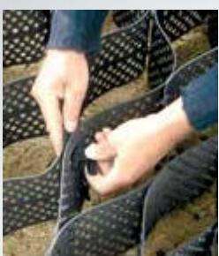
For quick and easy connection of GEOWEB sections, exclusive ATRA keys significantly reduce contractor installation time.
